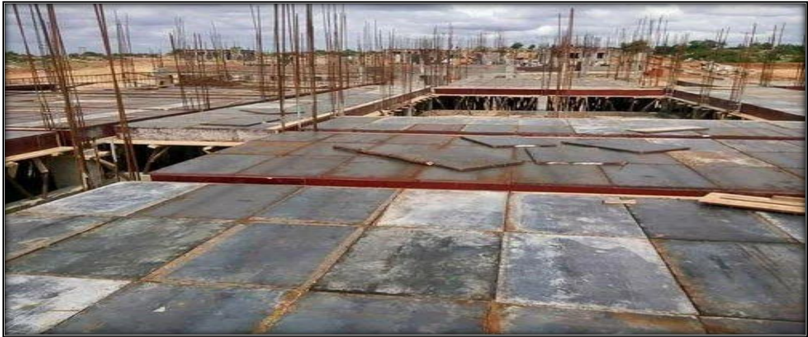
Figure 11: scaffolding, formwork and centering work.
